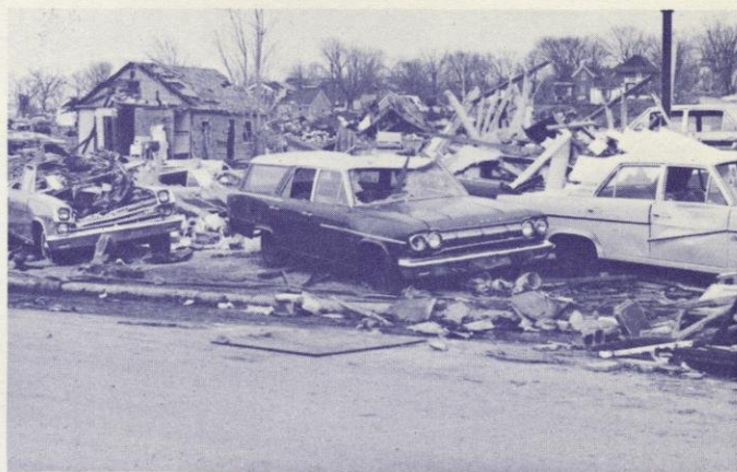
MONROE —Residential areas, such as above, took on the appearance of junk yards following the destructive storm.
