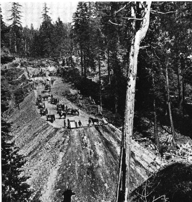
Chinese laborers use picks and donkey carts to make an 82 foot fill on the Central Pacific.
