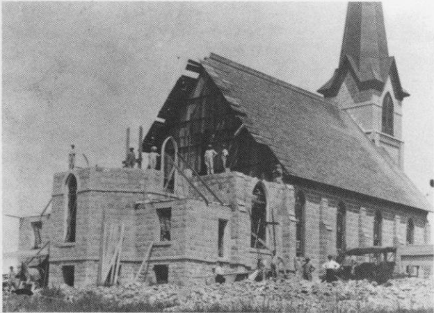
The stone being laid in this 1914 remodeling came from chief mason Erick Erickson's farm, 27 in the Sandy Rock School District.
