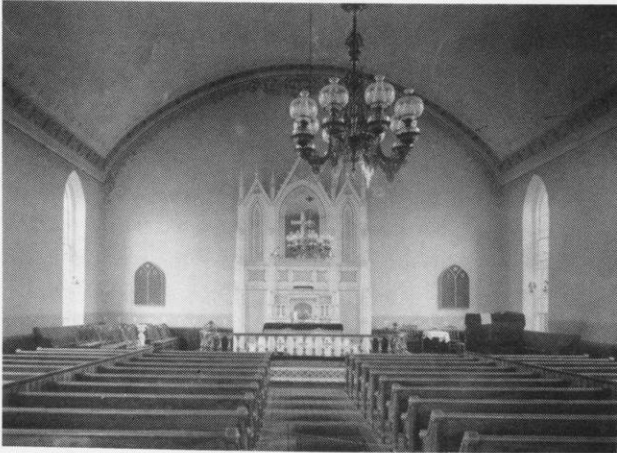
The interior of Perry Lutheran Church in 1881
