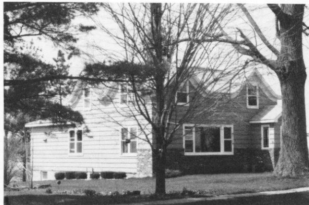
The house John Stensby built for his own family about 1900 as it looked in 1991 when Bennie and Verna Grundahl were living there.
