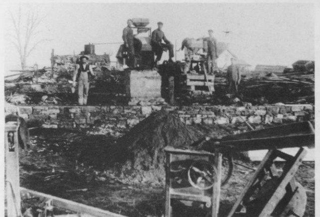
Building the Daleyville Creamery. The Daleyville Garage followed on this site.
