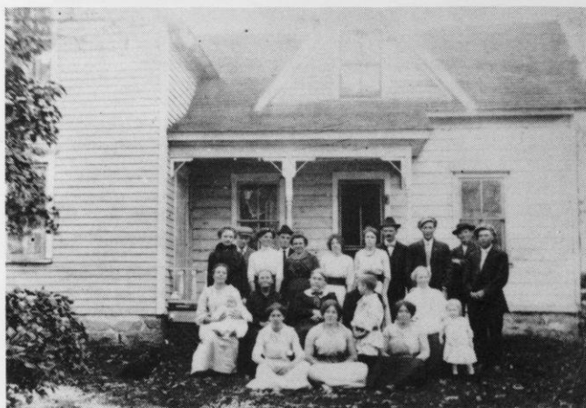
This was a one-story, one-room log cabin when the Olsons and Schlimgrens lived here. Gradually it was improved. The logs were covered with clapboard and a two-story addition was tacked onto one end of the cabin. This made the house L-shaped, with the original cabin serving as the one-story kitchen wing.
