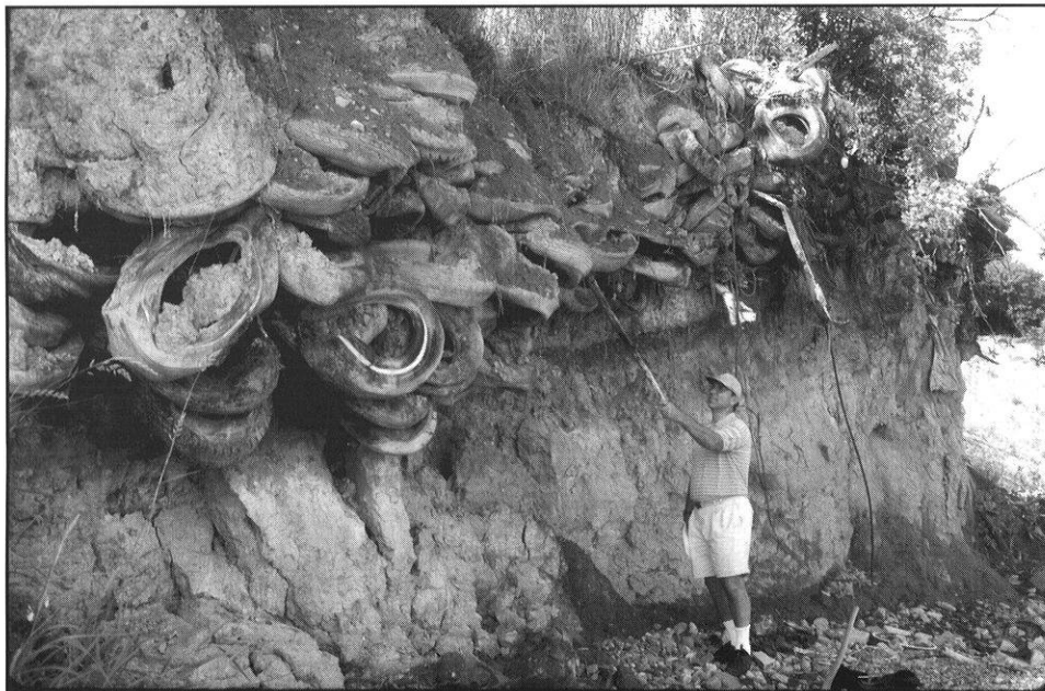
Professor Tuncer Edil examines some tires about to fall into Lake Erie due to bluff failure near Painesville, Ohio.
