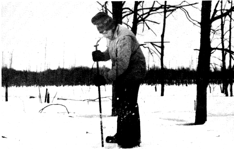
The first step is to insure that firm soil exists on the flowage or lake floor for pole placement (left). A hydraulic soil auger is then placed through the hole in the ice and drilling extends to a depth of 6 ft for a 30-ft pole (right).
