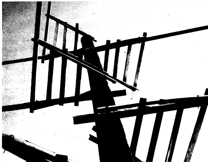
Platforms placed consecutively in 180° rotation are recommended. Platforms such as these have a projected life expectancy if new of 45 years, and if used, 15 to 20 years.
