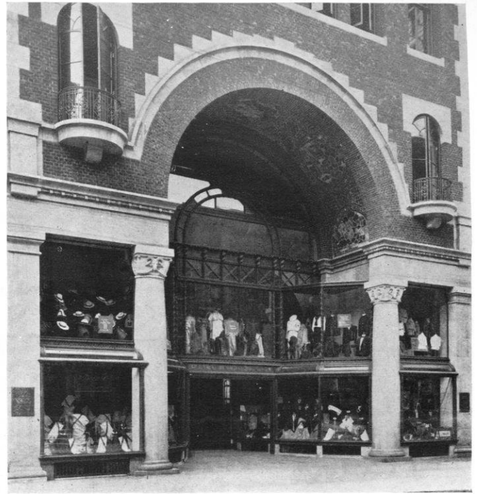
VIEWS OF STORE, CHESTNUT STREET, PHILADELPHIA: SOFFIT PORCH FACED WITH TILE MOSAICS DEPICTING THE CRAFT OF CLOTHES MAKING FROM THE SHEARING OF SHEEP TO THE CUTTING OF CLOTH: ALL ORNAMENT HAVING RELATION TO USE FOR WHICH BUILDING WAS DESIGNED: NOTE CAPS OF COLUMNS WITH CARVED RAMS' HEADS HOLDING GARLANDS OF WOOL, ALSO BOBBIN-REEL MOLDING.
