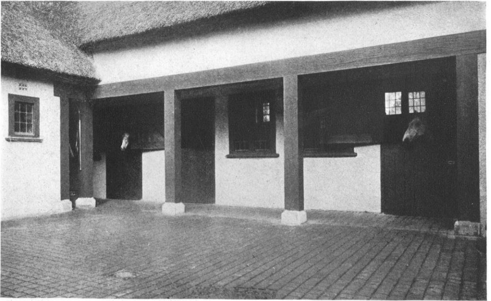
THE STABLES AT MINEHEAD, SHOWING LOOSE BOXES AND PAVED YARD.
