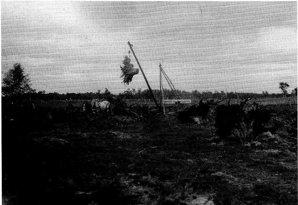
Figure 3. A Conrath piler lifting stumps onto a pile for burning. The team of horses provide the power to lift the stump. Courtesy State Historical Society of Wisconsin.
