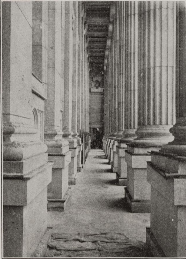
HARRY JOHNSON, General Contractor, Omaha, Nebraska.
