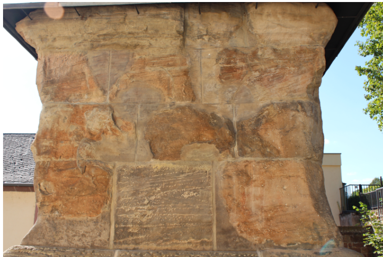
Figure 71: Badly damaged eastern base panel of the Igel Monument from Igel in Germany, Sandstone, Early to mid-3rd Century CE. Image by Morgan Lemmer-Webber, Creative Commons Attribution-Share Alike 4.0 International.
