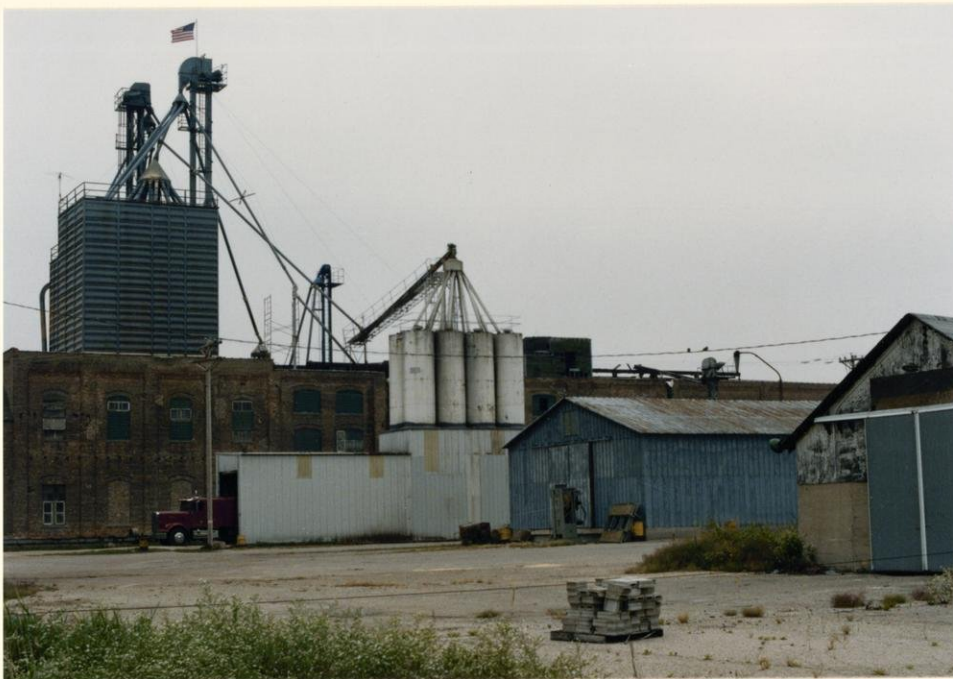
North side (back) of Garver main building showing grain elevator on roof, steel hopper building with truck in loading process, and corrugated steel warehouse - all owned by Garver. A warehouse owned by Madison Farm structures appears in foreground. Back of building is basically flat and unadorned. The architecturally interesting facade on the south side of the building is wasted due to the closure of Sugar Ave.
