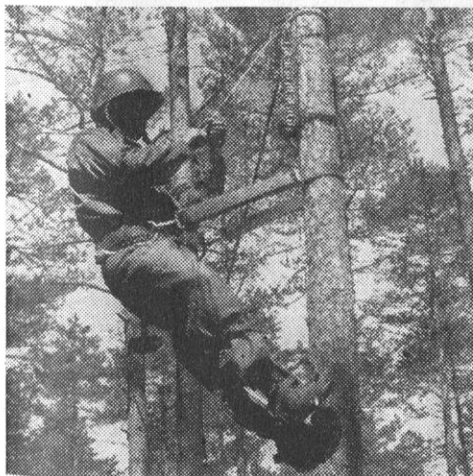
T/4 Robert L. Moyer, of the 1st Signal Company, 1st Infantry Division, works on the terminal strip of a field telephone.
