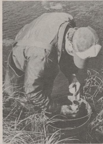
Collecting sediment taken from an irrigation ditch at a cranberry operation adjacent to Thunder Lake in Oneida County. The sample will be tested for heavy metals.
