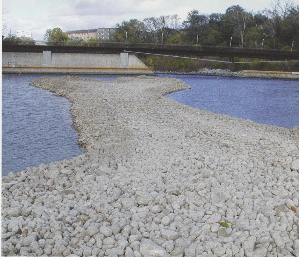
A walleye spawning reef has been created in the Milwaukee River Estuary. The reef stones needed to be small enough to attract walleye and other species to spawn but large enough to stay in place.
