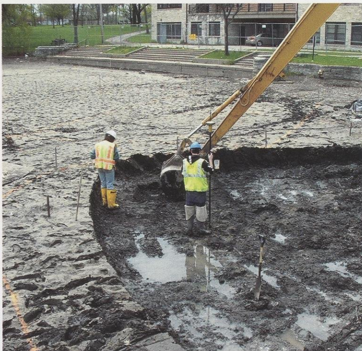
Sediment cleanup at the Blatz Pavilion lagoon removed about 300 pounds of PCBs in nearly 4,000 cubic yards of mud.
