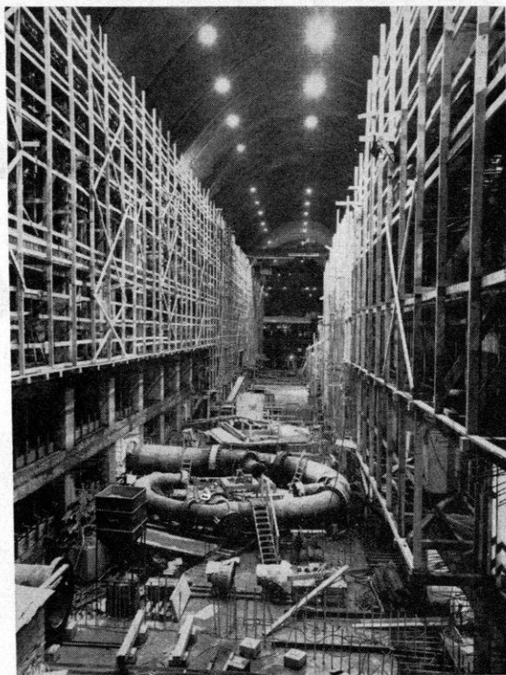
Tremendous problems were involved in building the 50-mile transmission line between Kemano and Kitimat, above. At right, a mammoth cave, all man-made, is the powerhouse and center of the B.C. project. The cavern is 700 feet long, 80 feet wide, and 118 feet high. It can be easily enlarged.
