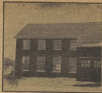
Front view of Pettit Apiary Building. Note the abundant provision for light, which makes inside work more attractive.
