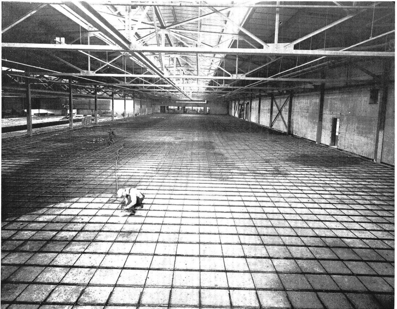
The warehouse for the Pacific Telephone and Telegraph Company, San Leandro, Calif., used more than 16,300 feet of corrosion-resistant wrought iron pipe to radiant heat 22,500 square feet of floor area. A wire mesh was stretched over the pipes to strengthen concrete "topping" slab and help to distribute the heat evenly. Mesh is then covered with 3 inches of concrete.
