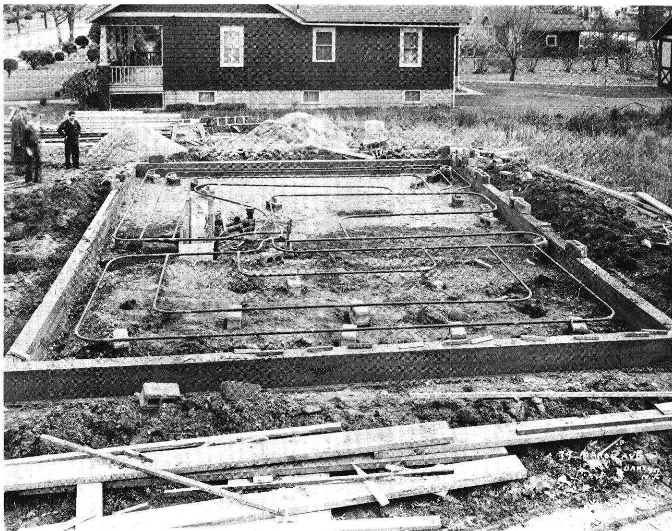
A residential wrought iron pipe radiant heating installation.
