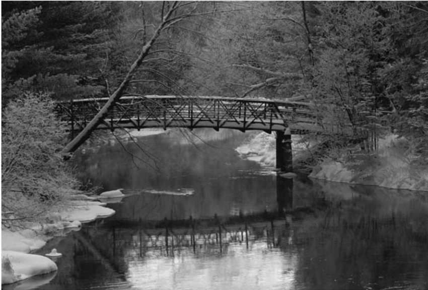
The Wayne E. Houghton Memorial Bridge is part of a snowmobile trail in Oneida County. There are approximately 24,000 miles of snowmobile trails in the state. (Department of Tourism)
