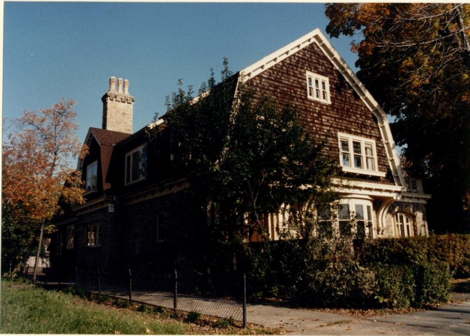
Northwest side of house--large open porch at main entry behind hedge. Note narrow driveway from Carroll Street to back parking area and carriage house.
