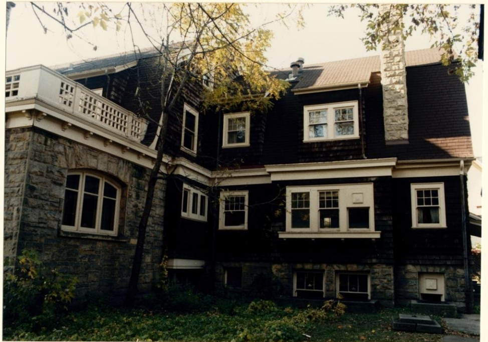
View of rear of house from open side yard. Three-season one-story porch at far left. Servants quarters on second floor and kitchen plus pantries on first floor. Basement area used for laundry and wine cellar. Portion of carriage house at far right.
