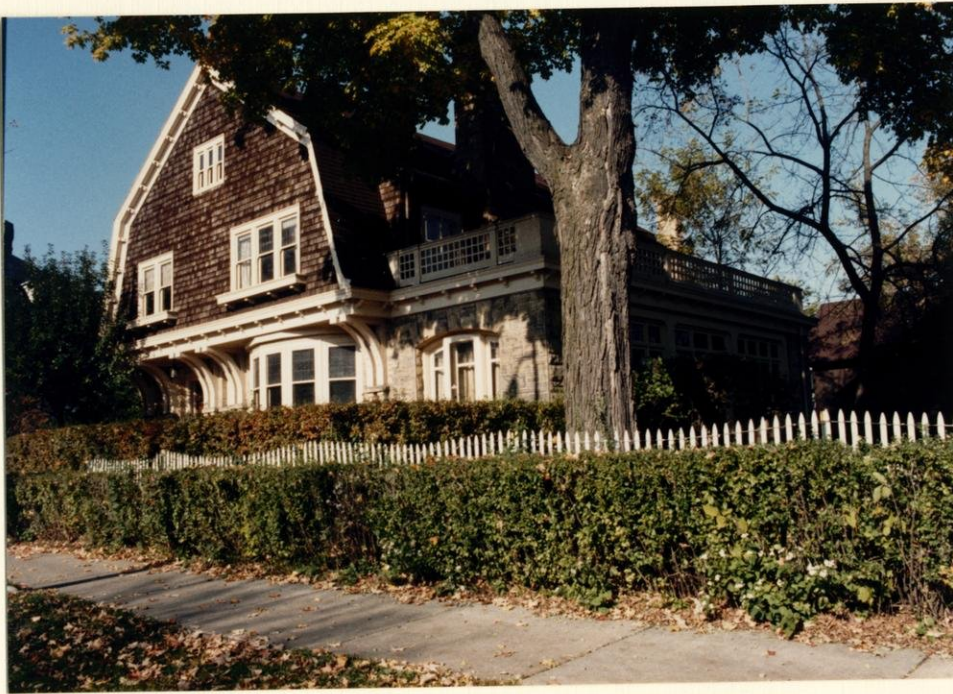
Looking north from North Carroll Street, main entry at far left of open porch. Note three-season porch with deck opening off main bedrooms on second floor. Carriage house in background at right.
