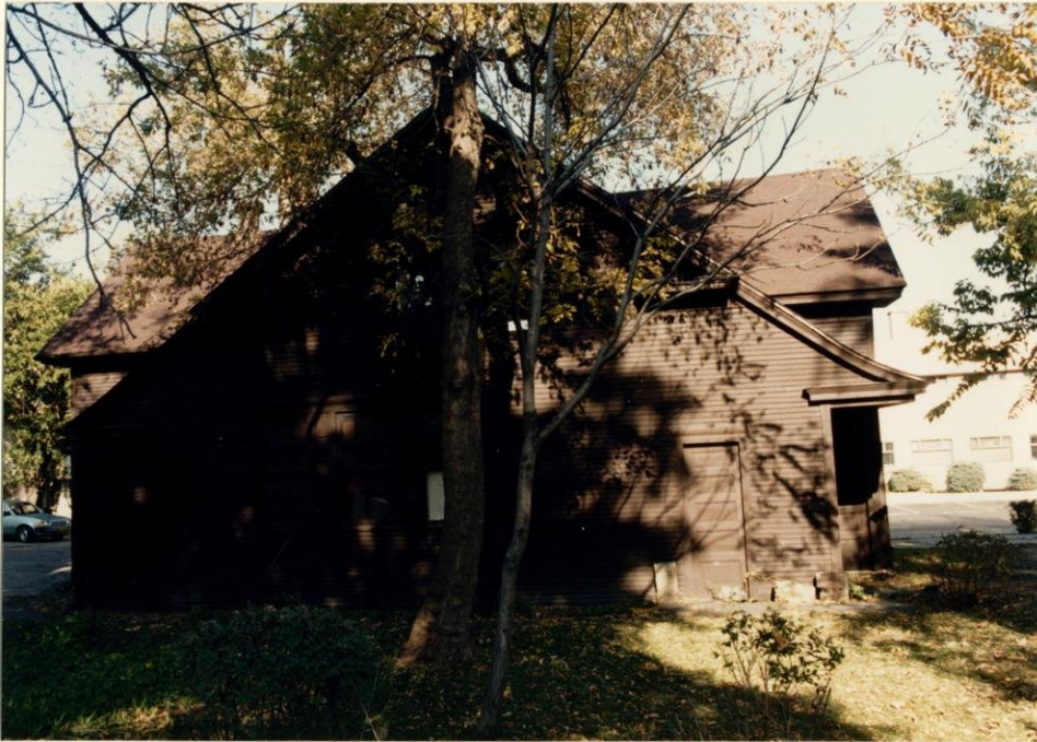
Carriage house as seen from open yard. Note paved area at far left on 415 North Carroll Street site.
