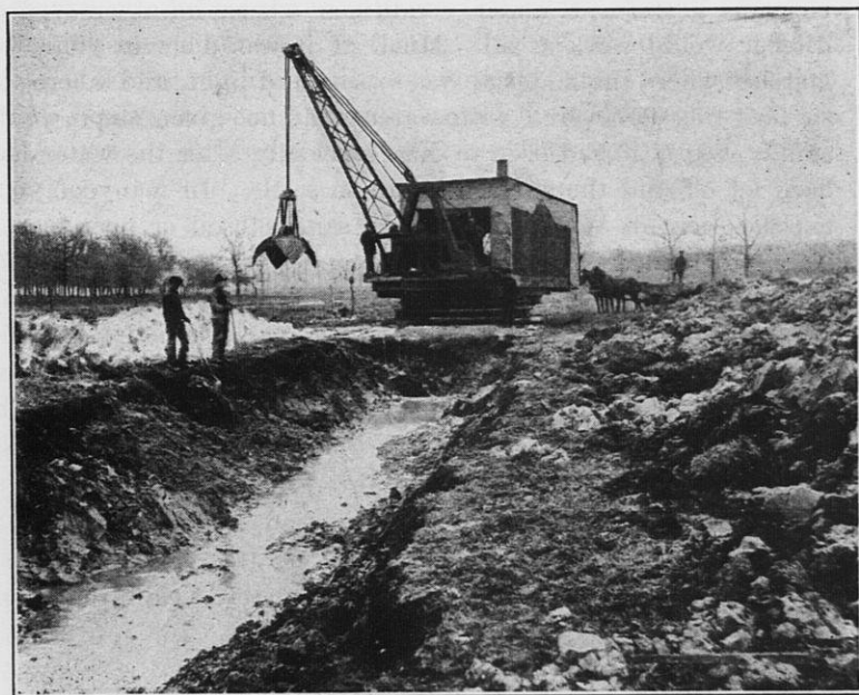
FIGURE 6.—A DITCH WITH A FAIR SLOPE.
