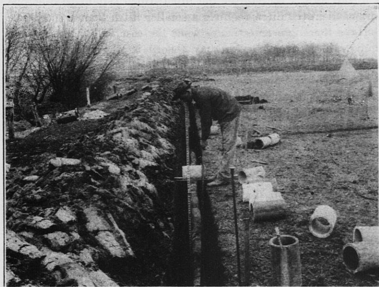
FIGURE 12.—LAYING TILE BY HAND.
