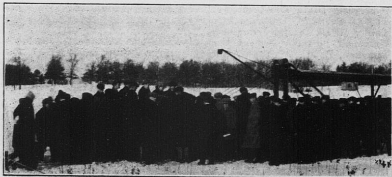
MANY WATCHED THE BUCKEYE MACHINE DIG A TRENCH IN FROZEN GROUND
