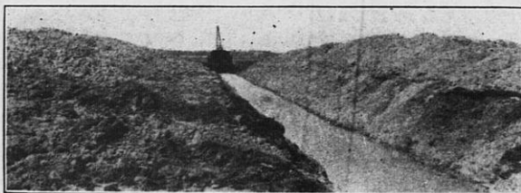
No. 1—T Monighan Walker excavating drainage ditch near Waterford, Wis.
