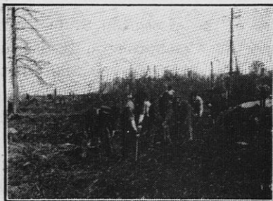
Making Holes for Blasting
