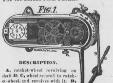
lever secured to shaft B: E. spring-
