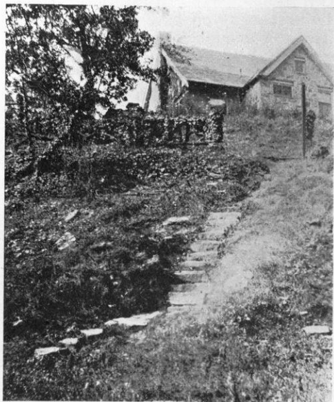
ROUGH STONE STEPS LIKE THE APPROACH TO AN ALPINE CHALET LEAD TO THE EAST WING OF THE HOUSE.
