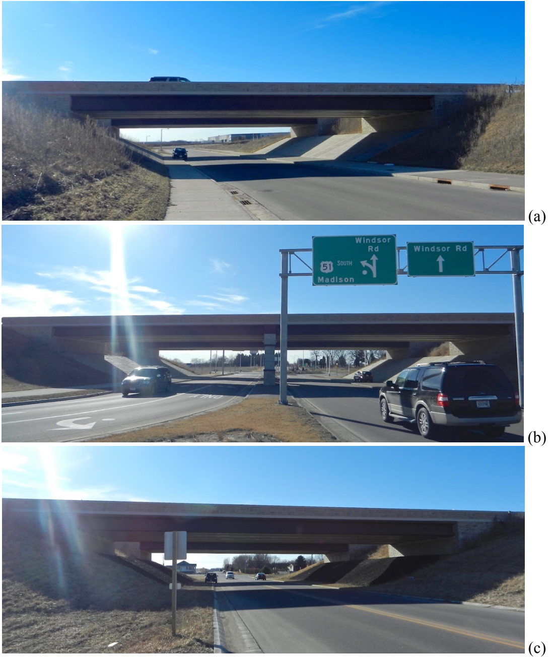
Figure 2.2. Pictures of the finished bridges on USH51: (a) Bridge over Bear Tree Road, (b) Bridge over Windsor Road, and (c) Bridge over Vinburn Road.
