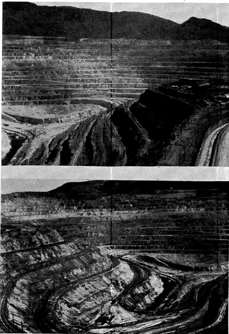
FIGURE 5.—Views of Chino mine, Kennecott Copper Corp., Chino Mines Division, Santa Rita, N. Mex., looking eastward
