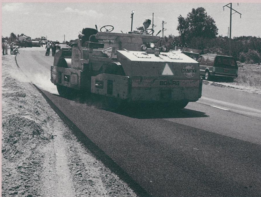
Where the rubber meets the road — recycled rubber is ground and mixed with asphalt in a paving experiment on Highway 12 in Eau Claire County. Photo by Dave Lyford
