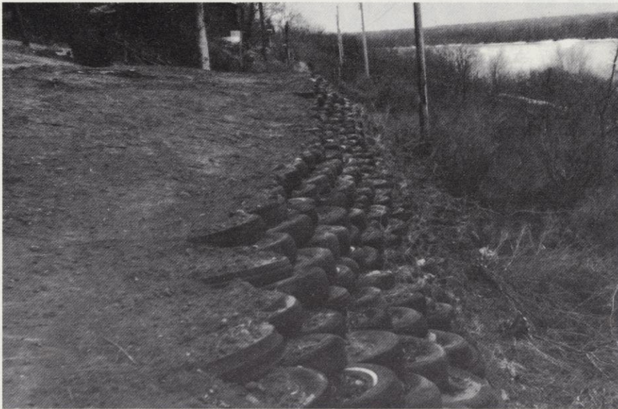
A tire embankment in Pierce County will be covered with soil and seeded with a quick-growing grass — voila, a berm! Photo by Dave Geister
