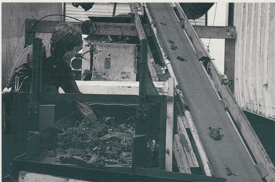
Shredded tires tumble down a conveyor belt at Winnebago Tire in Kewaskum. Larger chunks will be chopped again into two-inch pieces. The chips are sold for fuel in stoker-fired boilers.
