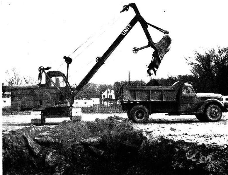
(Photo by Hull) The big day finally arrived. Here a power shovel is removing dirt for the basement of the new engineering building.
