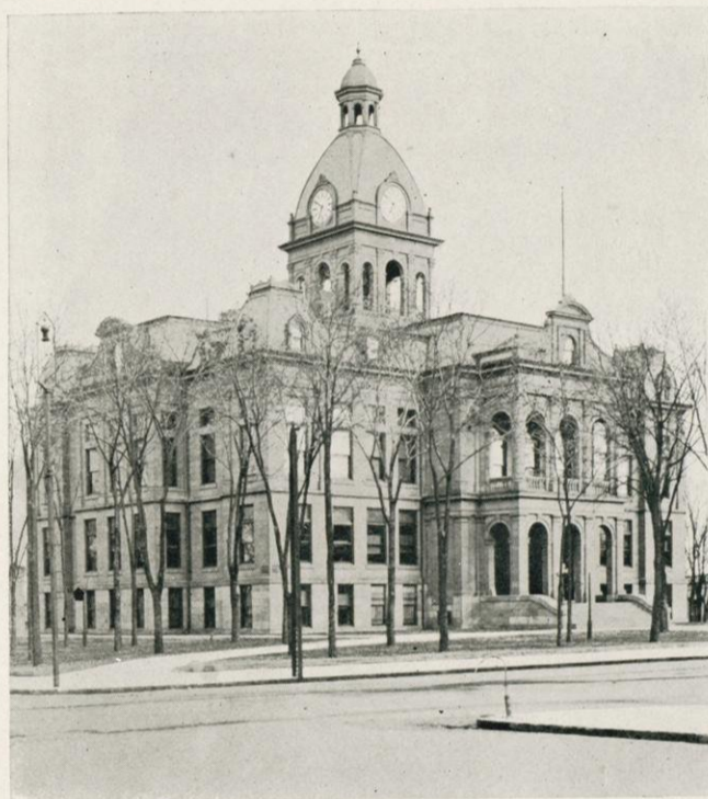
LA CROSSE COUNTY COURT HOUSE, LA CROSSE, WISCONSIN.
