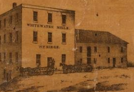
VIEW OF W. B. RIEGE'S MILL, WHITEWATER.
