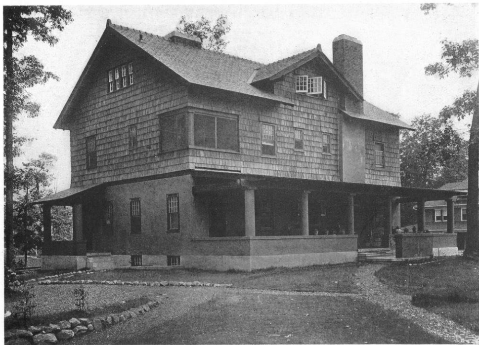
TWO VIEWS OF THE HOUSE OF MR. B. A. TAYLOR, BEECHWOOD PARK, SUMMIT, N. J., SHOWING ENTRANCE, AND LIVING PORCH AT THE SIDE.
