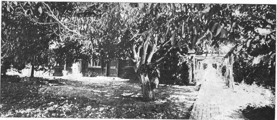
VIEW OF BUNGALOW HIDDEN IN WALNUT AND ORANGE TREES.
