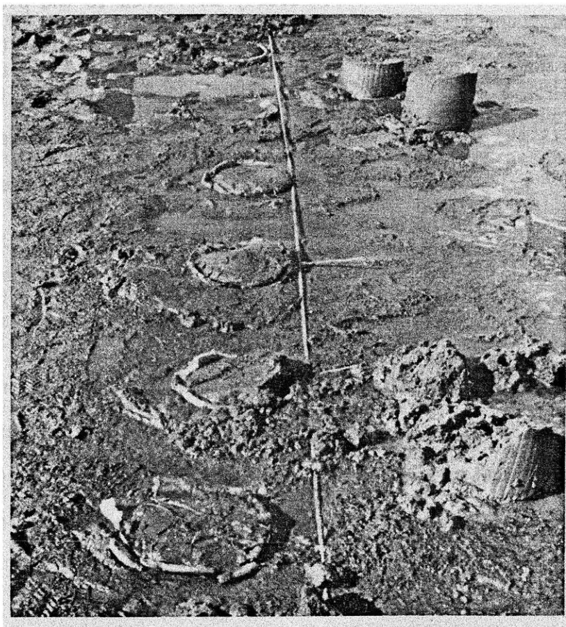
Figure 6. Potted plugs of Zostera planted at 0.6 m centers on intertidal dredge material at Site C (1978).
