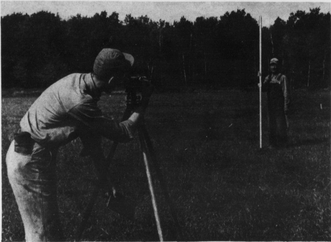
John Krzykowski, 18 Green Elm Club (Fifth year) (left), using level to stake out drainage type terrace. Joe Jagodzinski holding rod (right).
