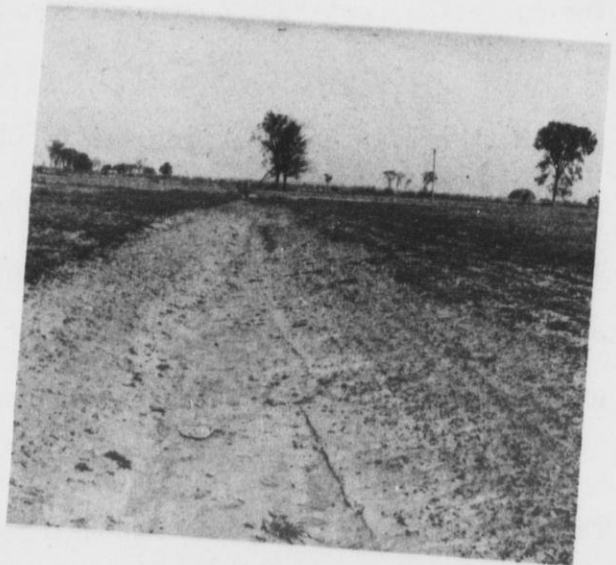
Cross section of water disposal ditch, George Otto farm, Rudolph town - cost $20.00 for 25 rods of ditch.
