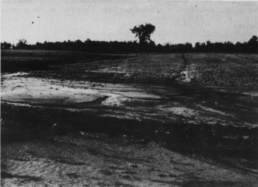
Serious sheet and gully erosion with fertile top soil deposited in foreground. Field has 2% slope.
