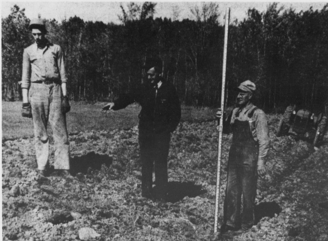
Cross section of drainage type terrace constructed with mold-board plow. Joe Jagodzinski farm, Sherry township.
