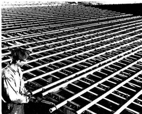
(photo courtesy Link Belt Co.) Figure 6
