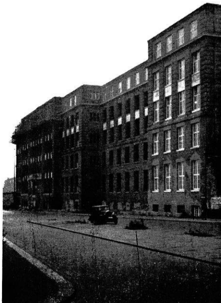
Main building which was bombed during the war. Reconstruction can be seen on the right wing and fifth floor.
