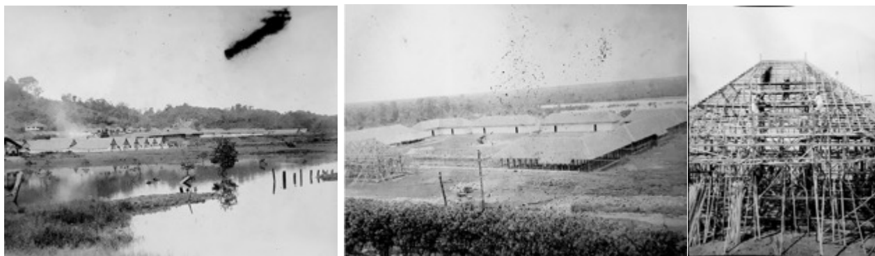
Figs. 3.6, 3.8, and 3.9: Prison facilities on Nusakambangan in 1925. Note in the above left image how the structures are temporary barracks with fabric roofs in the foreground, and permanent structures in the background. Towards the left, there is constant smoke coming from the rubber processing shed. The above center image is Batu Prison consisting of permanent structures constructed over the course of 1925. The upper right image shows prisoners constructing a building within Batu Prison.
