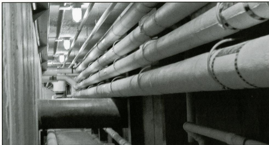
The pipe system underneath the Maquina Fountain extends across the length of Engineering Mall, supplying water to both fountains.
