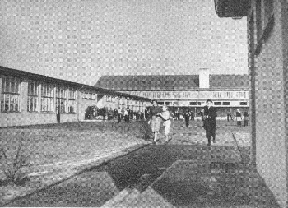
Left, partial view of Habenhausen Elementary School, one of five being built in Bremen to replace war losses. One third of all Bremen schools were destroyed in the war, which left only 20 percent of classroom space usable. The state of Bremen's school reform law is the most progressive in Western Germany. (Photos by Jacoby, PRD HICOG)
