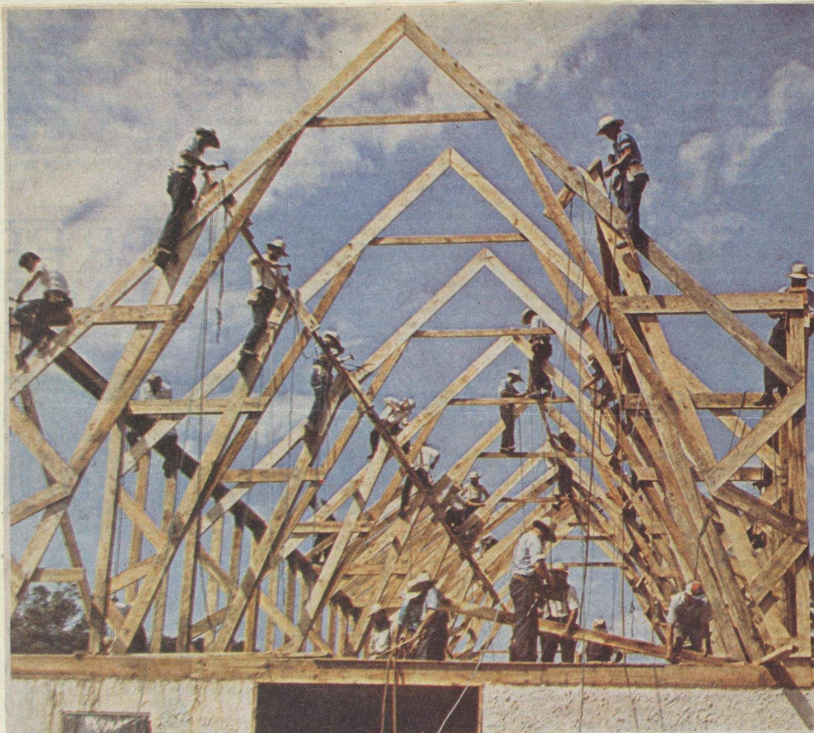
Stein — A scrambling 'army' hammers together the rafters of a new barn in Black Earth.
