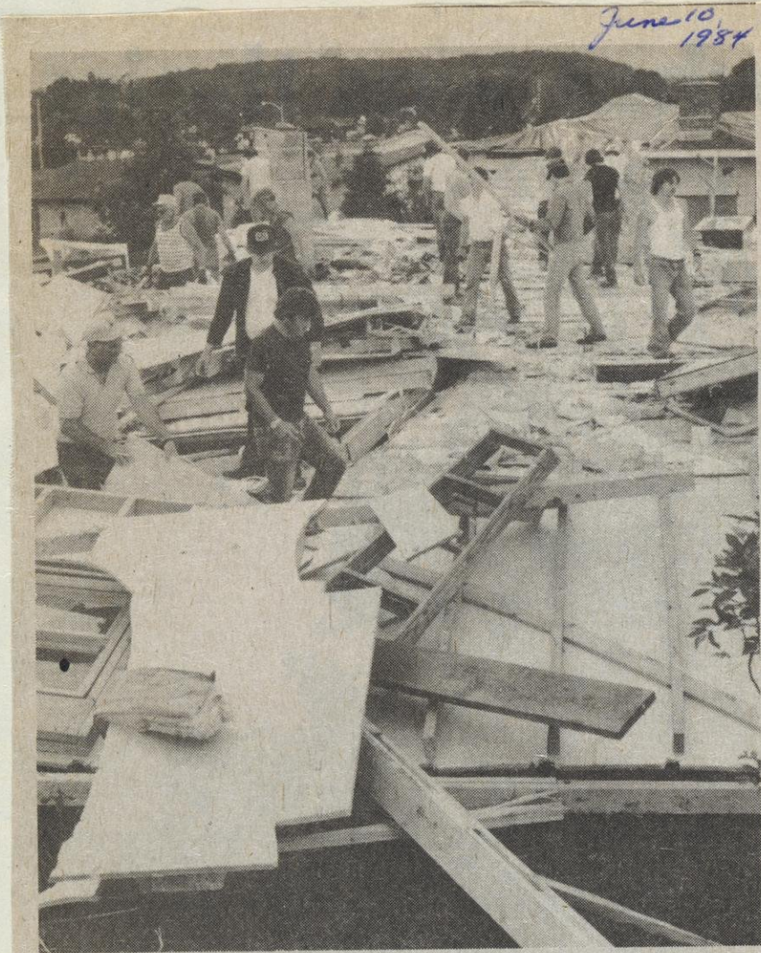
Black Earth residents walk through debris, assess damage.
