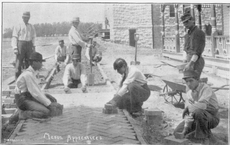
BRICK LAYING, HASKELL SCHOOL, LAWRENCE, KANS.
