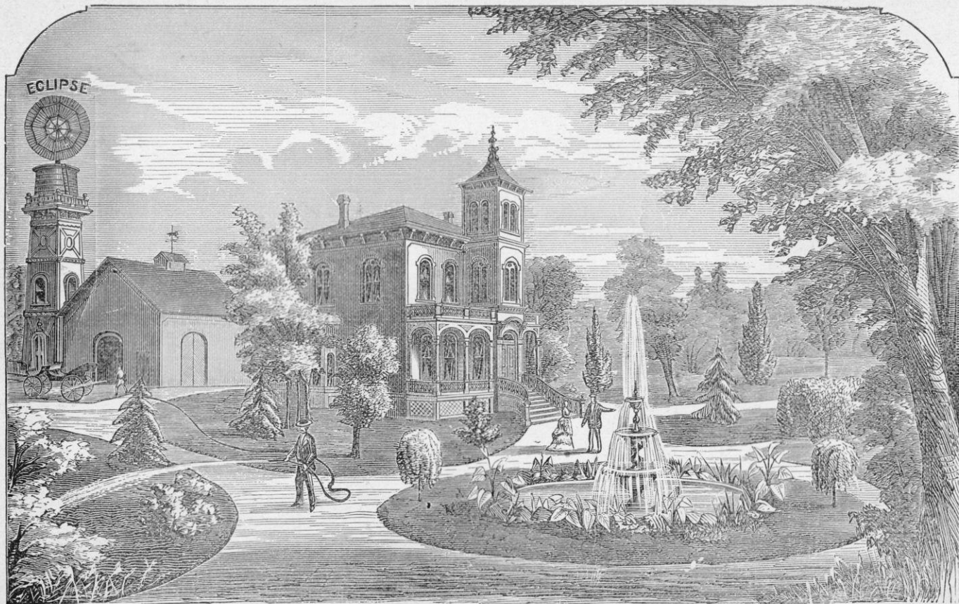
SUBURBAN WIND MILL WATER WORKS, AS ERECTED BY THE ECLIPSE WIND ENGINE CO., Beloit, Wis.
