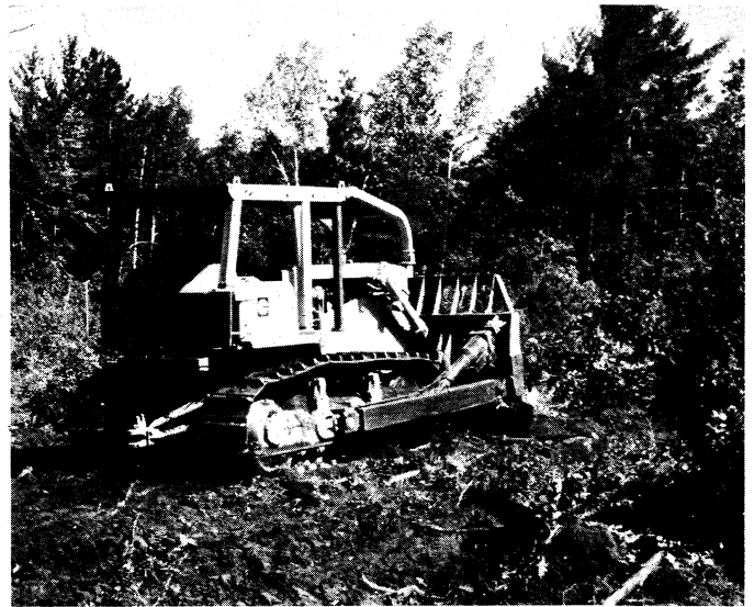
Openings were roughed-in by using a medium-sized dozer and a landclearing blade. This phase of construction was usually completed by private contractors.
