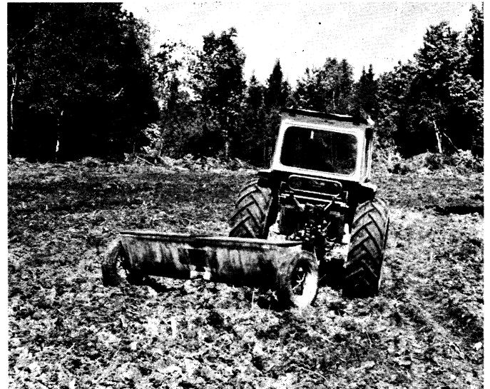
After leveling with a small dozer with blade and heavy disc, openings were fertilized and seeded using a wheeled tractor.
