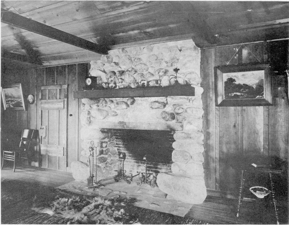
THE CHIMNEY PIECE IN THE DINING ROOM IS BUILT FROM GRANITE BOULDERS GATHERED FROM A DRIED-UP WATER COURSE NEARBY.
