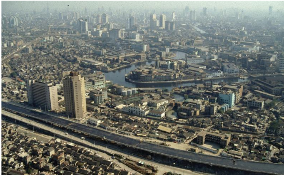
(The area where Dadi would be located in November 1998 before its construction)
