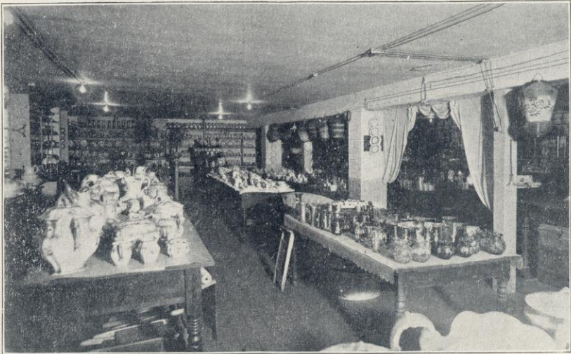
LOWELL HARDWARE CO. LARGEST RETAIL HARDWARE STORE IN WISCONSIN.
