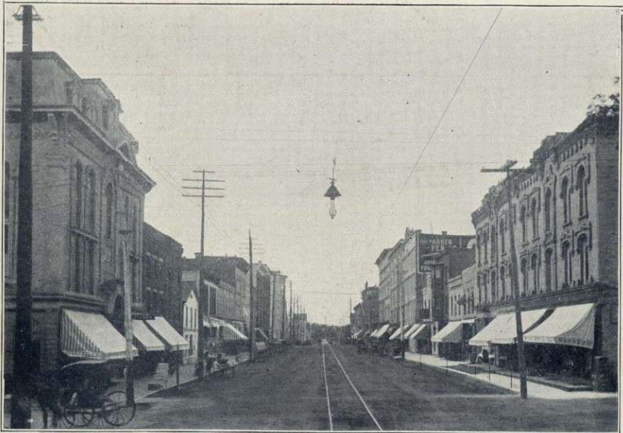
MAIN STREET, LOOKING NORTH FROM COURT STREET.
