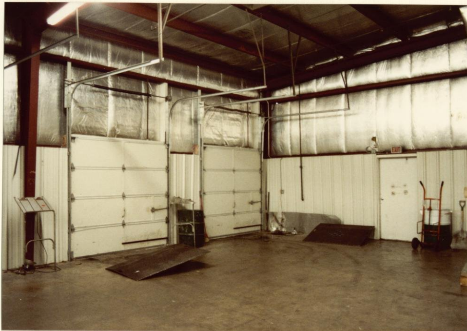
Northeast corner of Murphy Motor Freight Lines at 2201 Darwin Road. Note insulation, wall finish, and dock doors.
