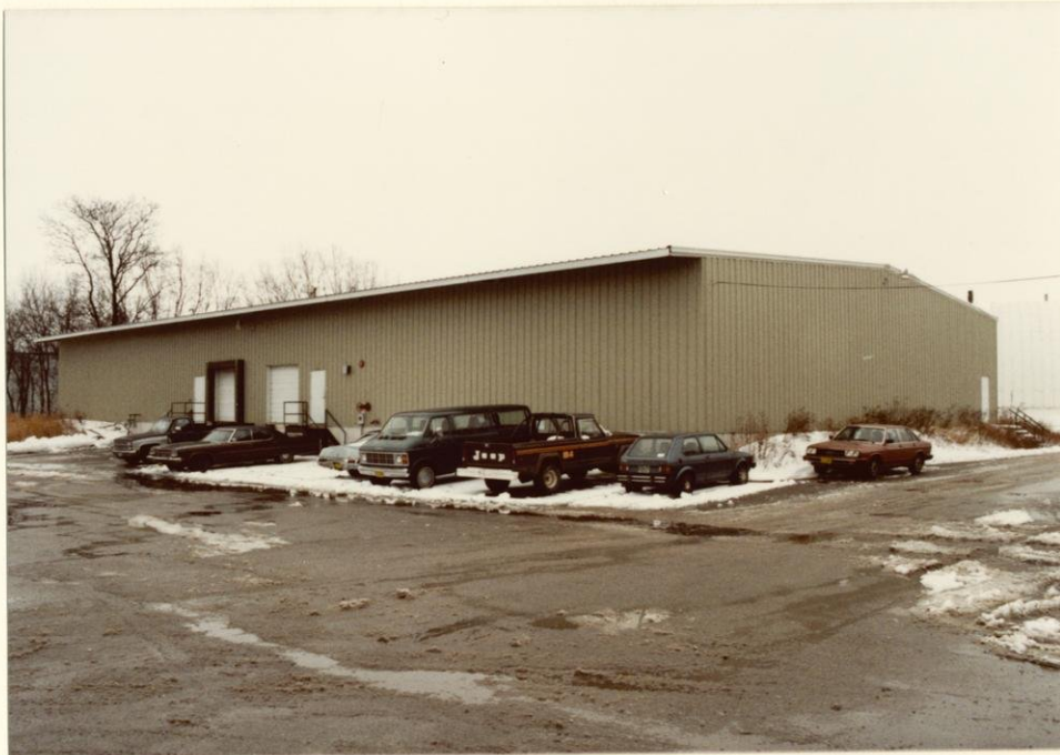
North side of 2223 Darwin Road. Note location of two dock doors and two personnel doors which makes division of building to suit two tenants feasible.
