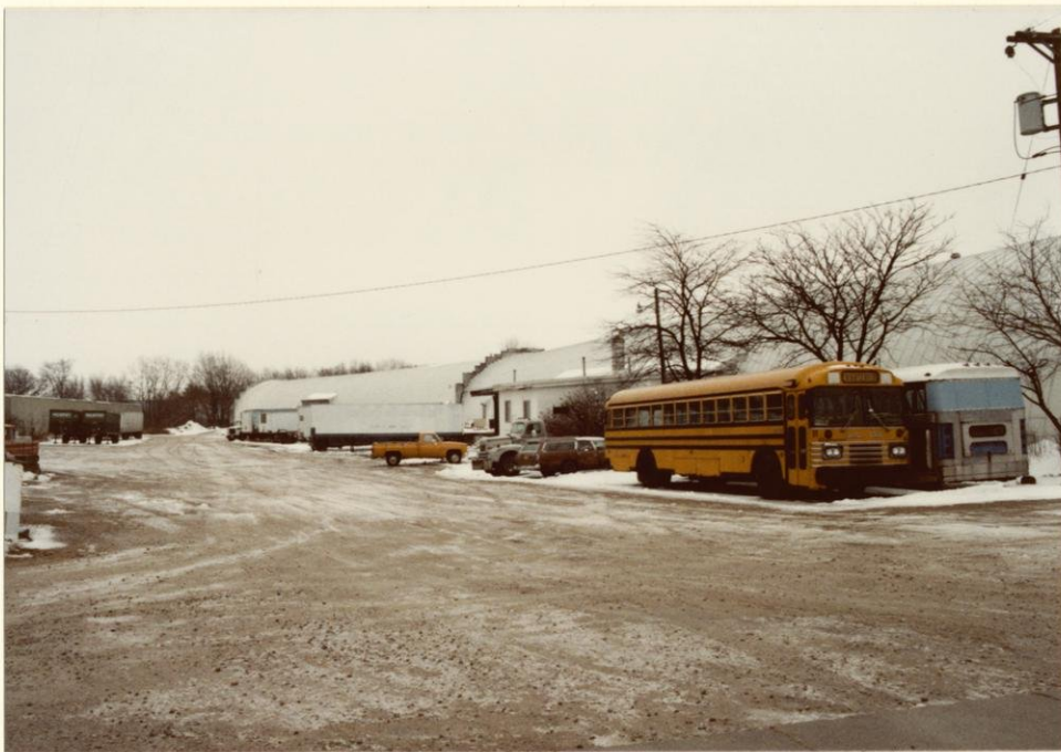
Length of quonset warehouse. Note concrete block firewall midway, just beyond office and loading dock extensions.
