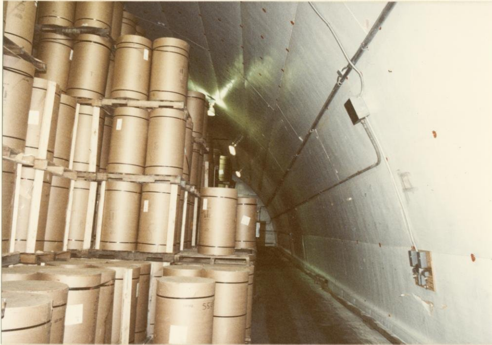
Interior of front half of 2955 Packers Avenue used for cold storage of surplus cheese. Note removable insulation installed by tenant and note number of pallets per stack.
