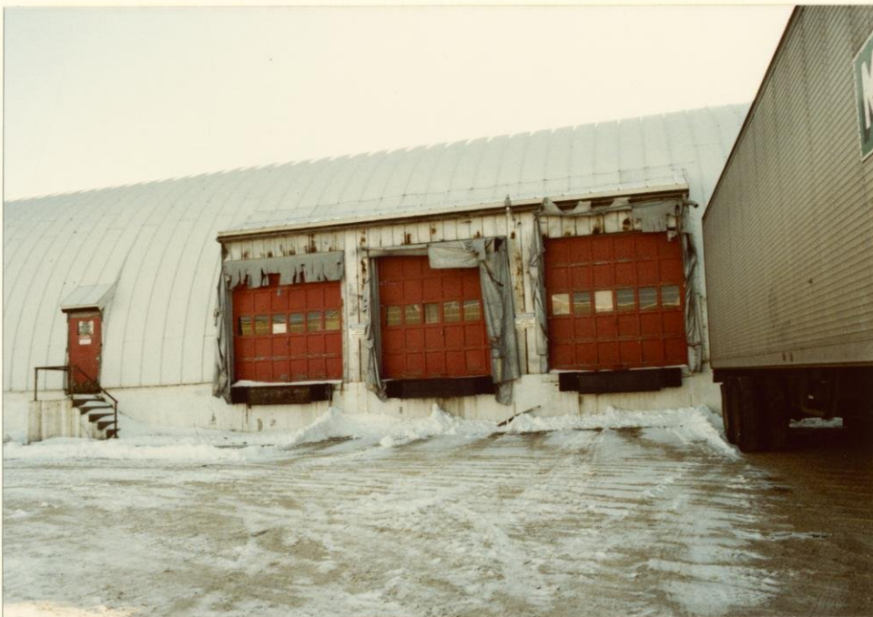
Truck docks on north side of east half of quonset warehouse at 2955 Packers Avenue.
