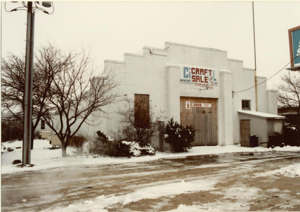
Front of quonset warehouse facing 2955 Packers Avenue. Note old overhead door and window boarded shut for cold storage operation.
