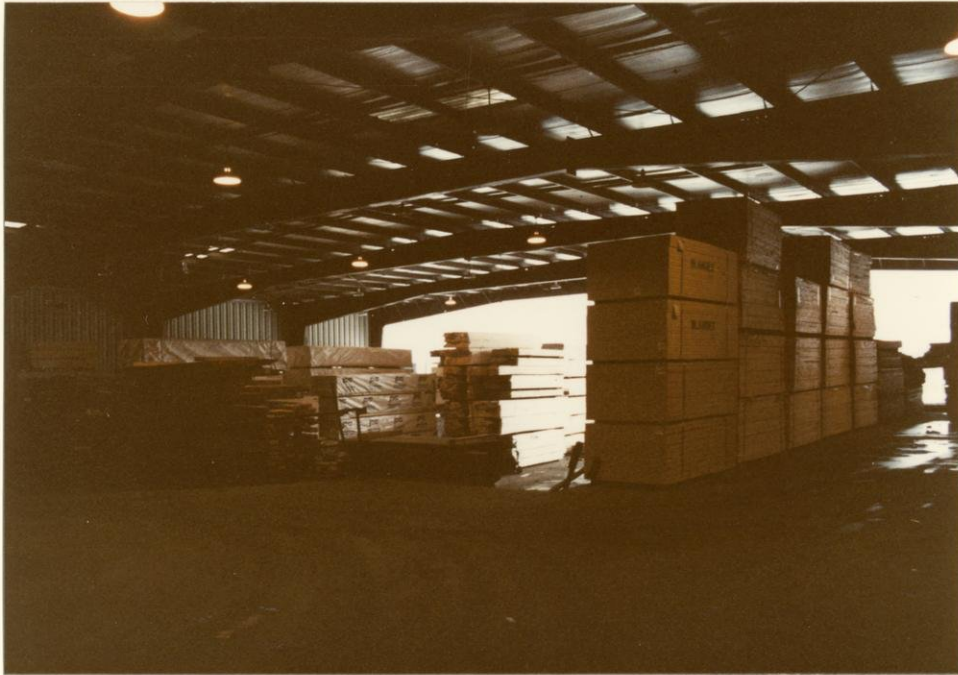
Looking east from top of ramp and dock inside open shed.
