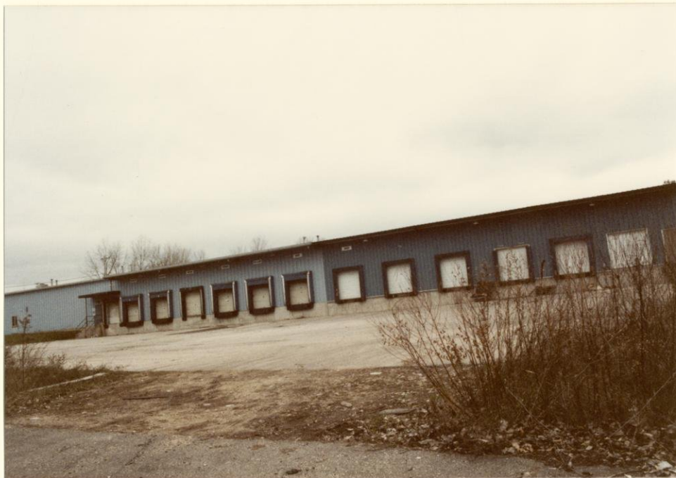
South side of warehouse at 2601 Seiferth Avenue. Darker shade of blue denotes newer 1976 addition. Excessive number of docks especially designed for Prange Department Stores which used warehouse as regional distribution center.
