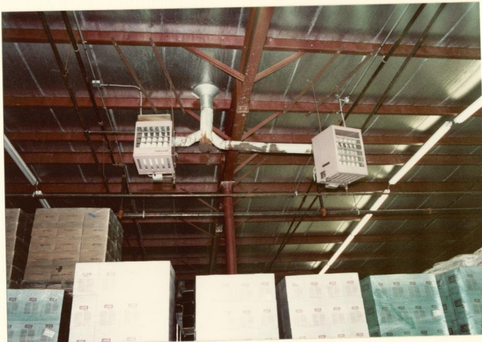
Interior space leased by single tenant, Delta Storage, at 2223 Darwin Road for storage of agricultural chemicals. Note suspended gas-fired space heaters. Interior finish similar to Delta Storage space at 2201 Darwin Road.
