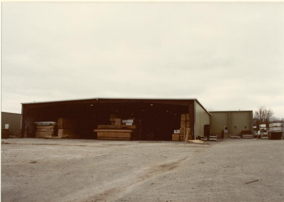
Open shed on east side of 625 Mayfair Avenue. Entrance to office area on far right of picture near west end of shed.
