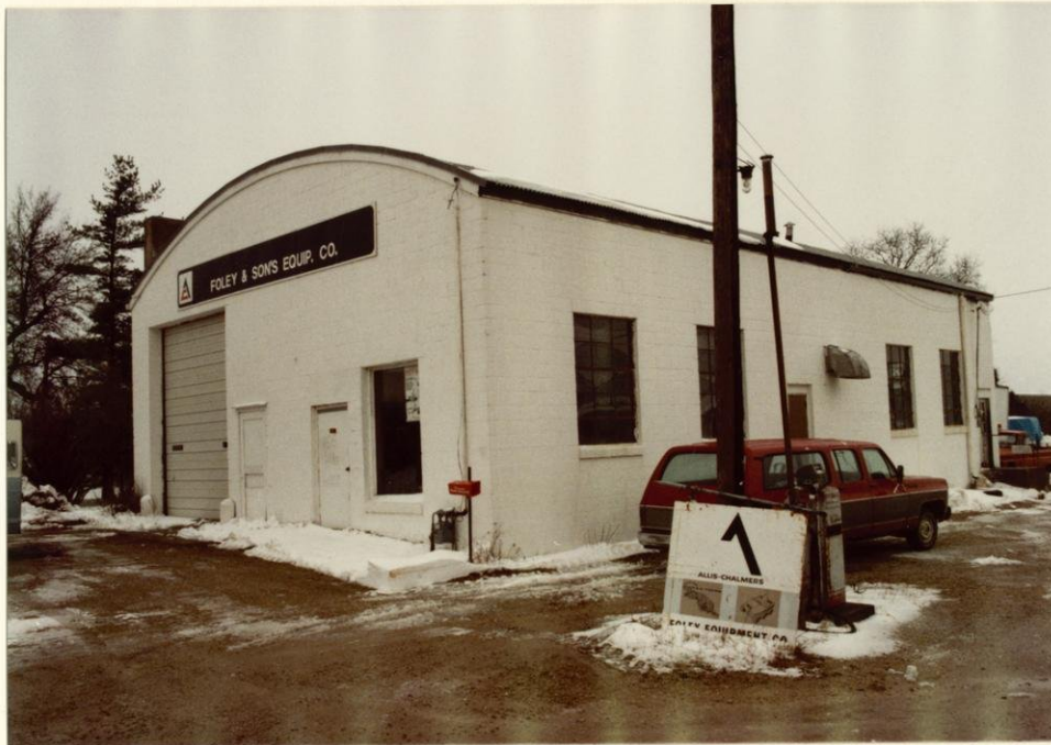
Concrete block service garage located on subject site at 2957 Packers Avenue. Note new overhead door at west end of building. Similar door also at east end of building.
