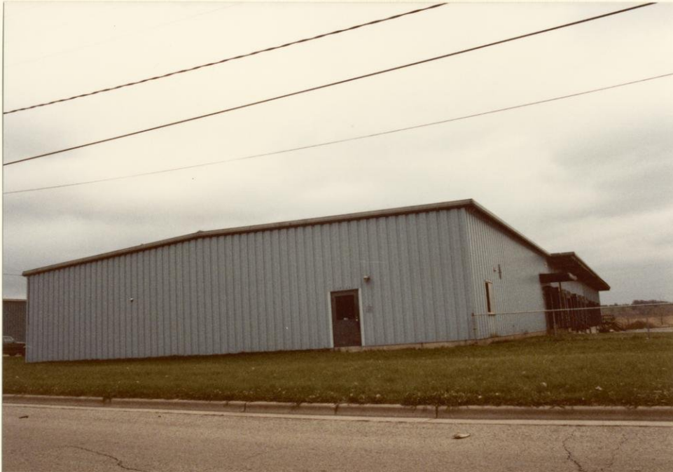
Looking east from Seiferth Road. Personnel door leads to unused office area.
