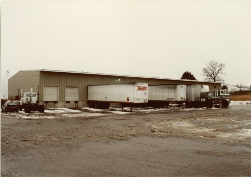
North side of 2201 Darwin Road with docks for Murphy Motor Freight at east end and Delta Storage at west end of warehouse. Note rail for handicapped ramp attached to east wall.
