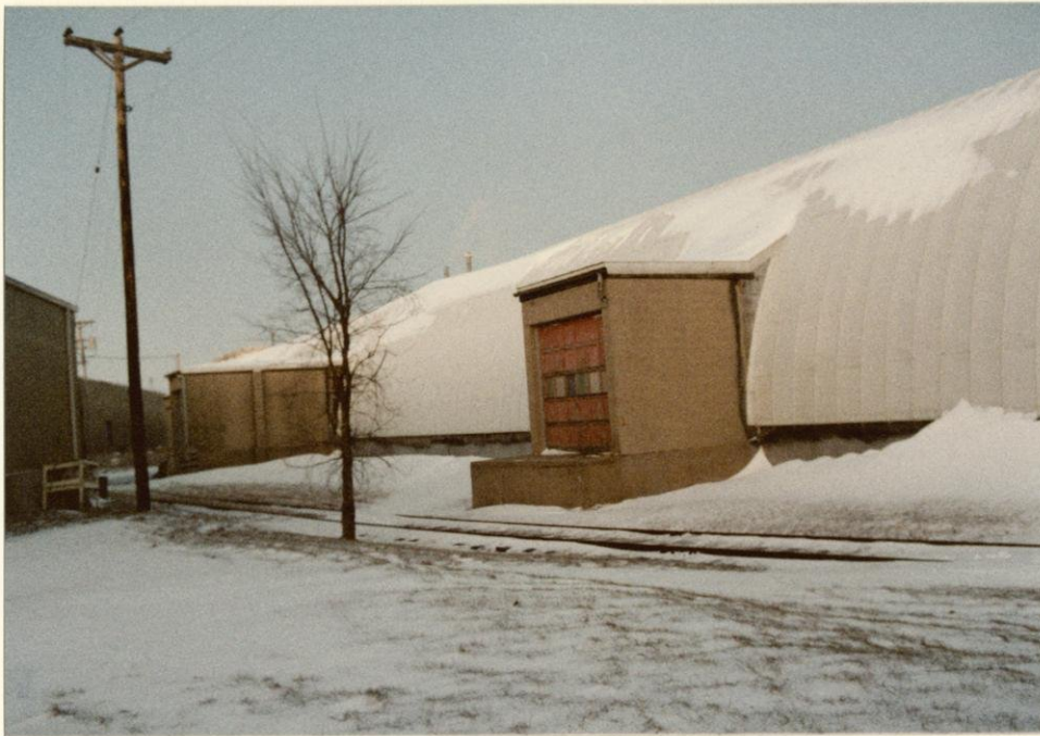
Rail docks on south side of east half of quonset warehouse at 2955 Packers Avenue
