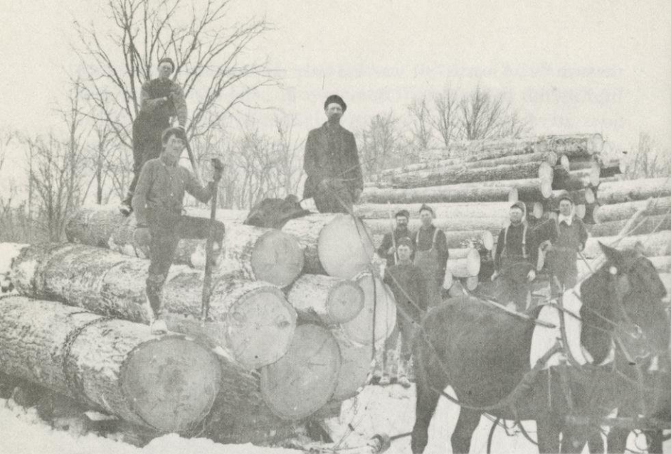
Hauling logs with horses, Necedah, Wis., about 1890. Below, hauling logs by sled. This load was built up for the photo. One team could pull such a load on the ice roads. Sometimes a lead team helped to get the load started. Photos courtesy of State Historical Society of Wisconsin.
