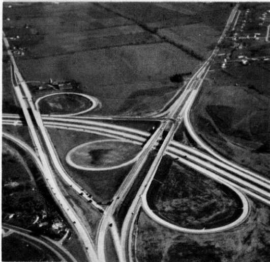
Important changes in the regional transportation system are encouraging urban expansion into the Fox River basin and thereby are directly and indirectly affecting the demand upon the resources of the Fox River basin. The effects of high standard highway facilities on the runoff characteristics and flow regimen as well as on the land use pattern of a watershed are readily apparent from this view of a new interchange recently completed in the upper reaches of the Fox River Watershed.
