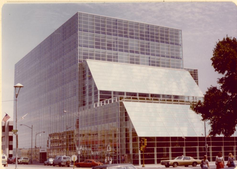
View to southeast of E. Washington Ave. facade from intersection of E. Washington and Pinckney
