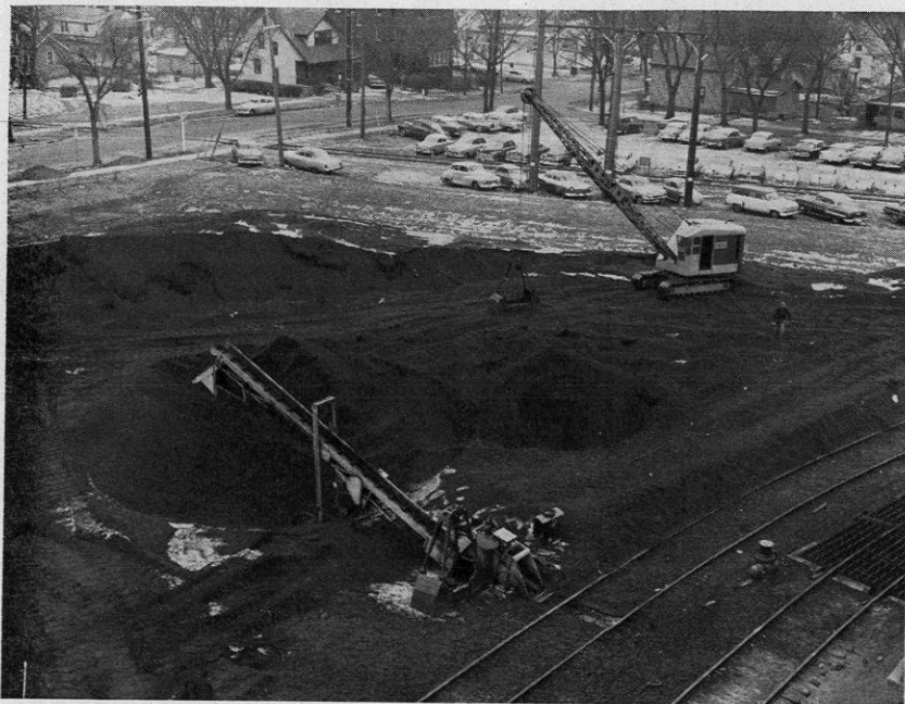
The coal storage pile with track unloader (left) and track hopper (lower right). Nearly 15,000 tons will be in storage when the stockpile is filled to capacity.
