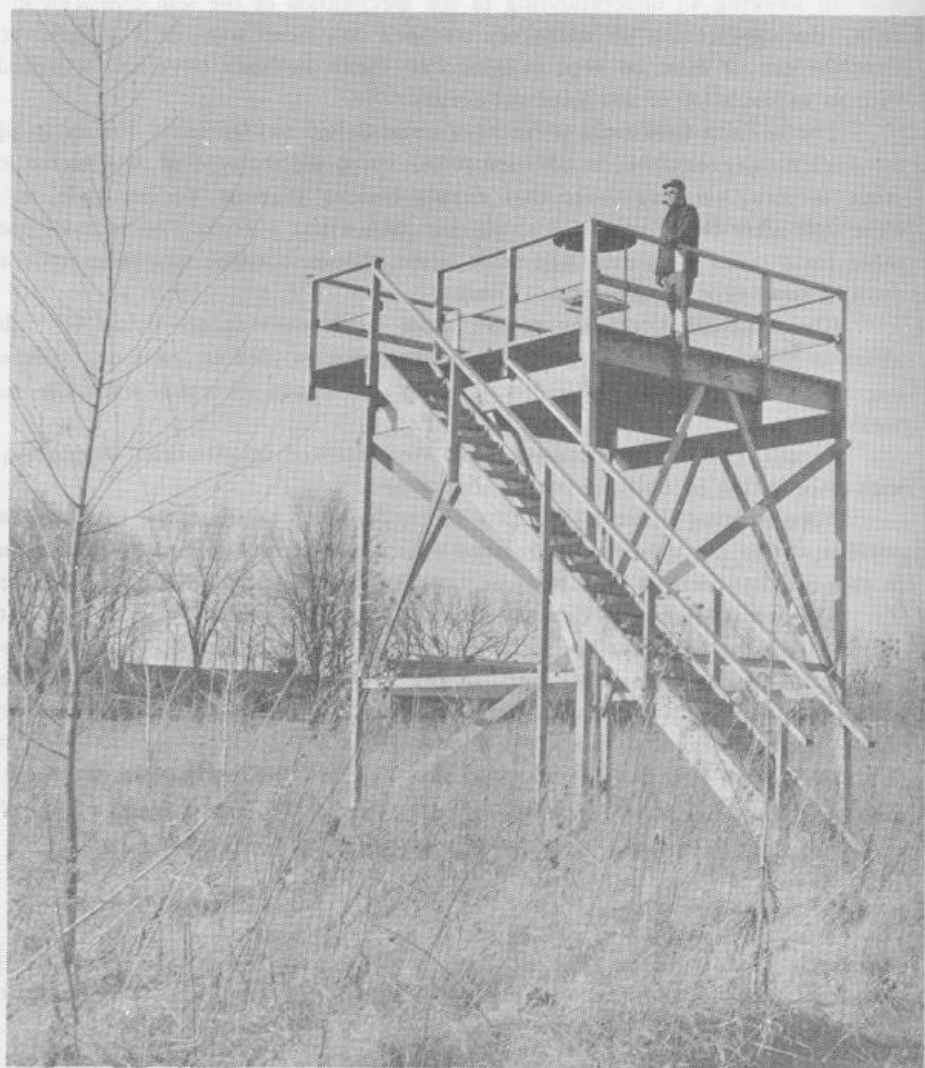
Fig. 1 Platform and tank erected immediately east of the headquarters. It is used in fish orientation studies.
