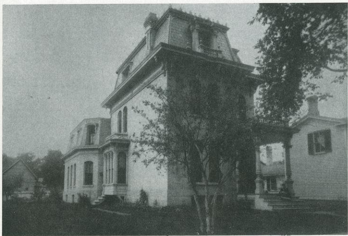
James Harris house, 170 S. Jackson, 1870. Photograph 1888. The high-styled residence of this Janesville industrialist was crowned by an ornate mansard roof.
