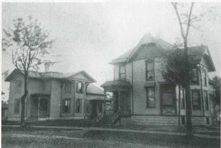
159 and 165 South Jackson. Photograph 1888. The two houses shown here are representative of the stylish Queen Anne houses built in the Old Fourth Ward in the 1880s. Asymmetrical plans, the combined use of clapboards and shingles, and ornate porches are typical features of the style. (From Picturesque Janesville Illustrated, 1888.)
