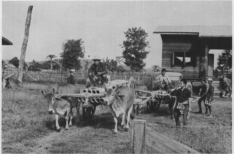
Transporting pipe to be used in a village water supply
