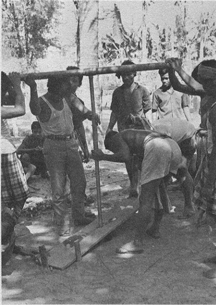
Using a hand auger to drill test holes for shallow wells
