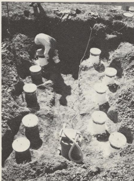
The "crust test" measures reduced water absorption in soil. Each pedestal marked a place on the ground surface run over by a back hoe. The spot was then excavated and a record made of the time it took for water to seep through the pedestal. The more passes by the backhoe, the lower the rate of infiltration. Photo by Jerry Tyler
