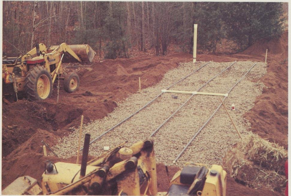
A mound system under construction. Photo by Jerry Tyler
